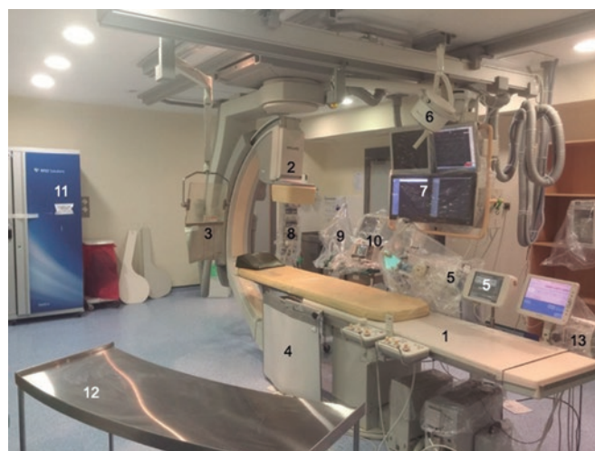
Figure 2. Equipment present at the cath lab. 1: patient table. 2: x-ray tube. 3: radiation shielding lead glass with upper leaded glass section and articulated adjustable arm mounted on the ceiling. 4: leaded skirt mounted on the table. 5: automated contrast media injector. 6: on/off ceiling light with adjustable articulated arm. 7: monitors. 8: infusion pumps. 9: anesthetic and respiratory equipment. 10: crash cart or code cart with defibrillator. 11: smart cabinet for material storage with automatic replacement. 12: table with the equipment needed to perform the procedure. 13: console of the pressure wire.
